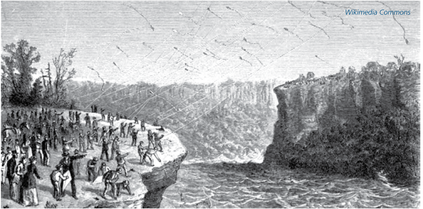
Engraving of the kite-flying competition that laid the foundations (cable) to build the Niagara Falls Suspension Bridge. Date: circa 1883
